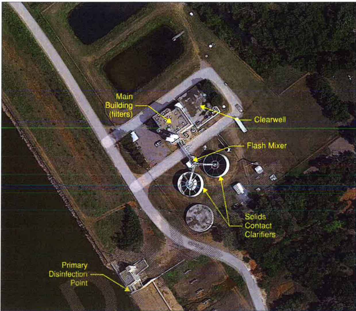
Figure 3-1: Aerial Image of Clinton Lake WTP
